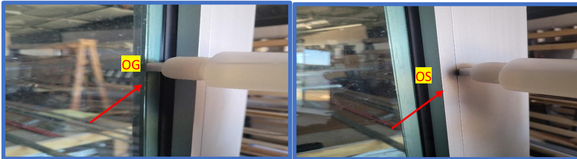
Figure 3. Example of Primer Application
